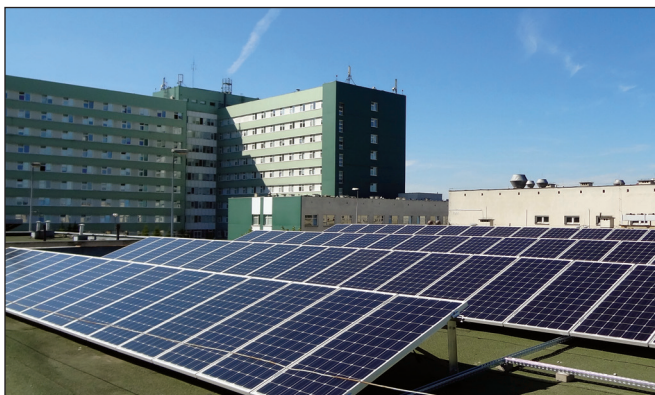
System PV w Radomiu o mocy 21 kWp
